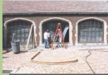
Workers install doors with Richards-Wilcox hinges in the historically accurate original design.
