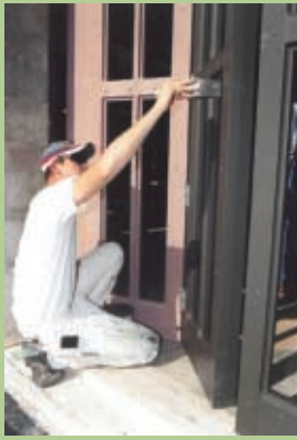
Workers install doors with Richards-Wilcox hinges in the historically accurate original design.
